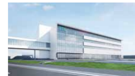
Kumamoto New Development Building (Completion scheduled for fall 2024)
