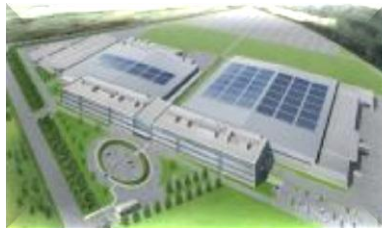
New Miyagi Plant
