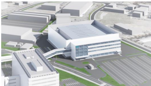
Koshi-city, Kumamoto Prefecture Completion scheduled for summer 2025
