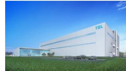
Tohoku plant: approx. ¥13.0B construction cost (Begin construction in October 2018, completion scheduled for September 2019)
