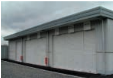
Waste storage facility (Koshi Plant)
