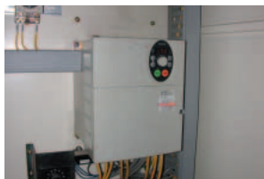
▲ Installation of inverters
