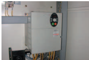
▲ Installation of inverters
