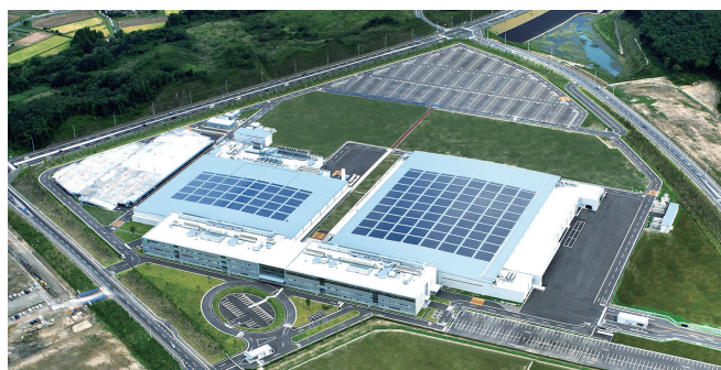
Tokyo Electron Miyagi Limited Head Office
