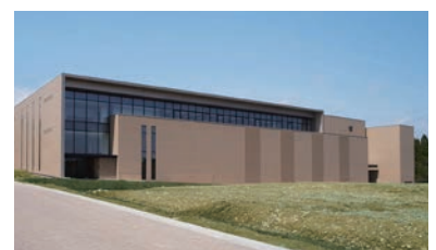
Tohoku University, Center for Innovative Integrated Electronics Systems (CIES)
